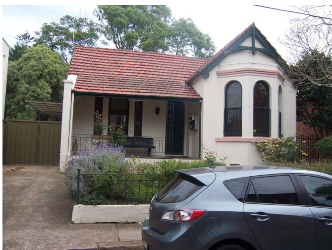
Photo 25. 10 College Street existing college use, zoned R2
