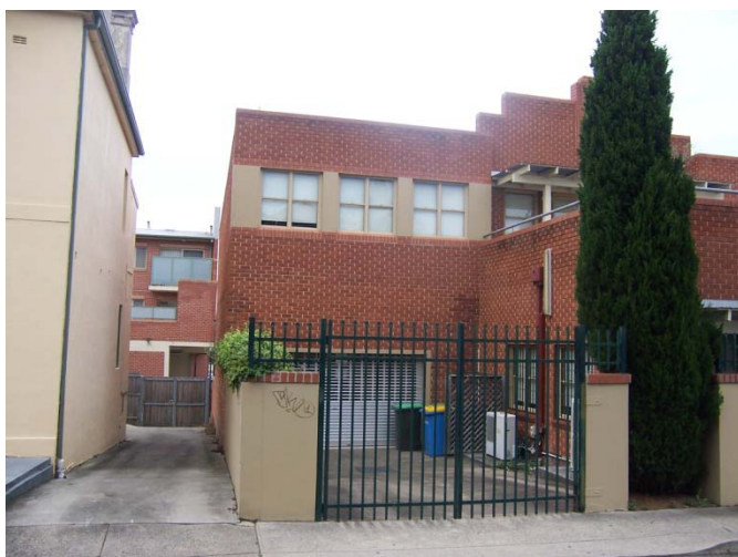
Photo 5, Rear of "The Croydon" , 11 College Street to left , a dwelling all zoned B2.
