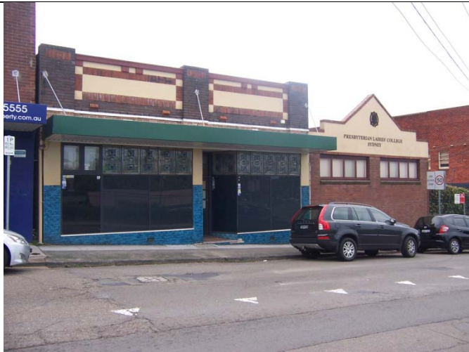
Photo 1, Existing college 2 College Street from Hennessey Street: zoned B2
